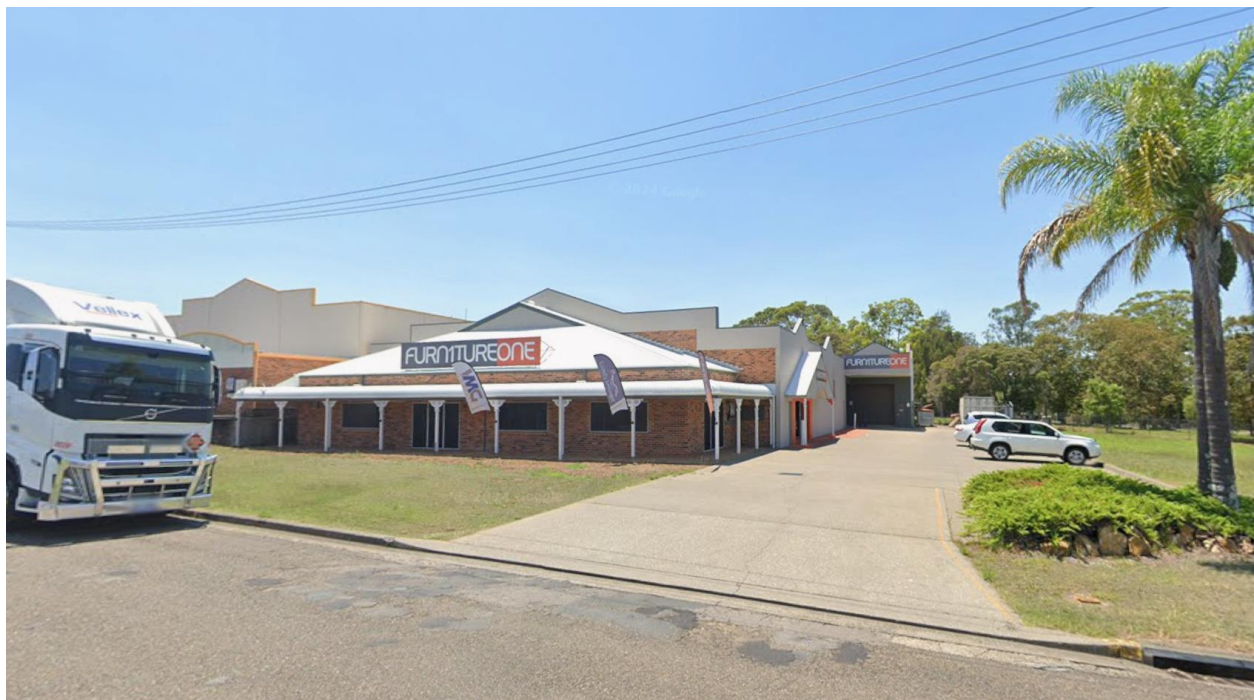
PHOTO 3: LOOKING EAST FROM MILL CLOSE TO SITES ACROSS THE ROAD
